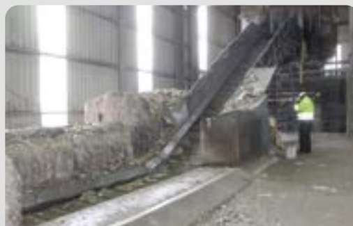
Infeed conveyors for recycled plastics
